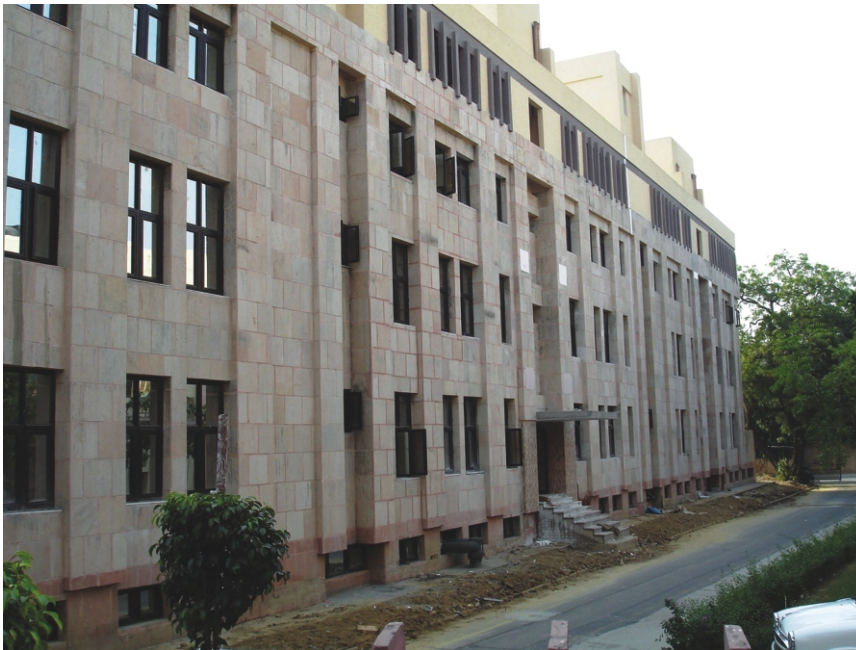
Delhi High Court Medical & Health Centre (Under Construction)
